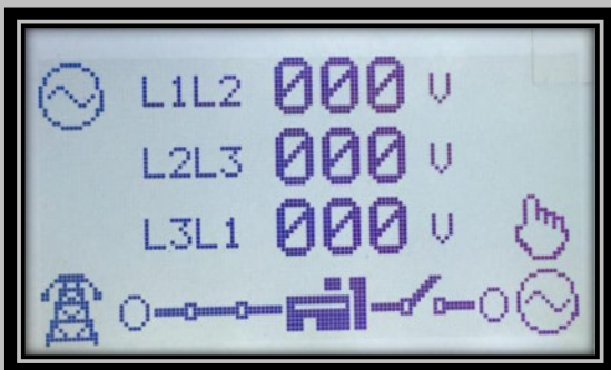
Generator Voltage ( L-L )
